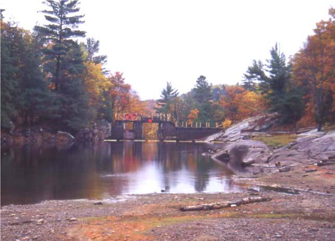
Figure 2. Redstone Lake dam with stoplogs removed. The water level is closer to the natural pre-dam level.
